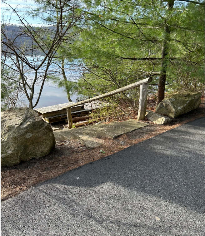
Similar cedar wood handrail at a Tuxedo Park property
