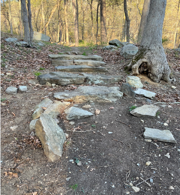
Existing condition/north entrance steps
