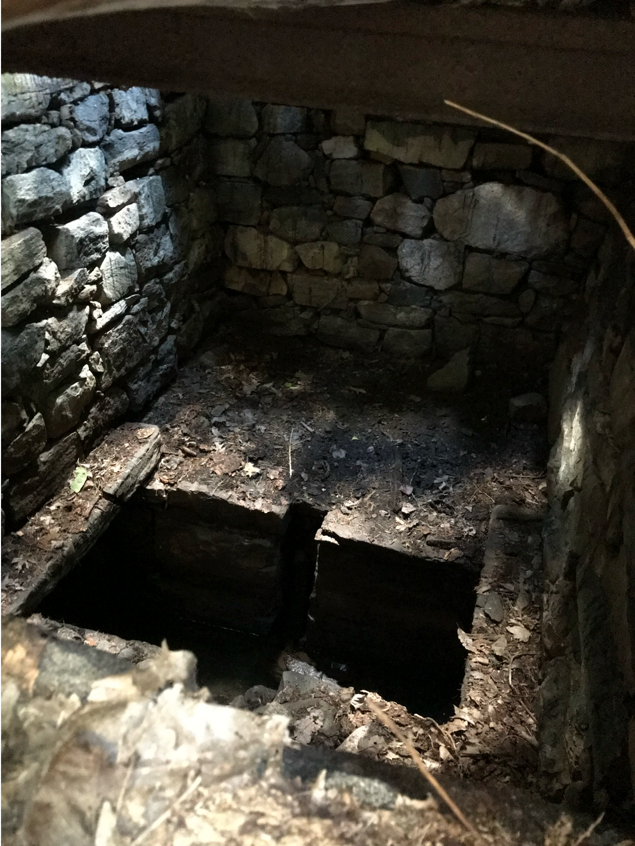
Interior of elephant drain: first level approx. 15' deep, second level another 15'?
