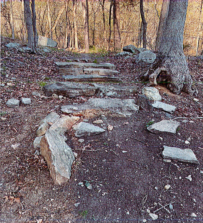
Existing condition/north entrance steps
