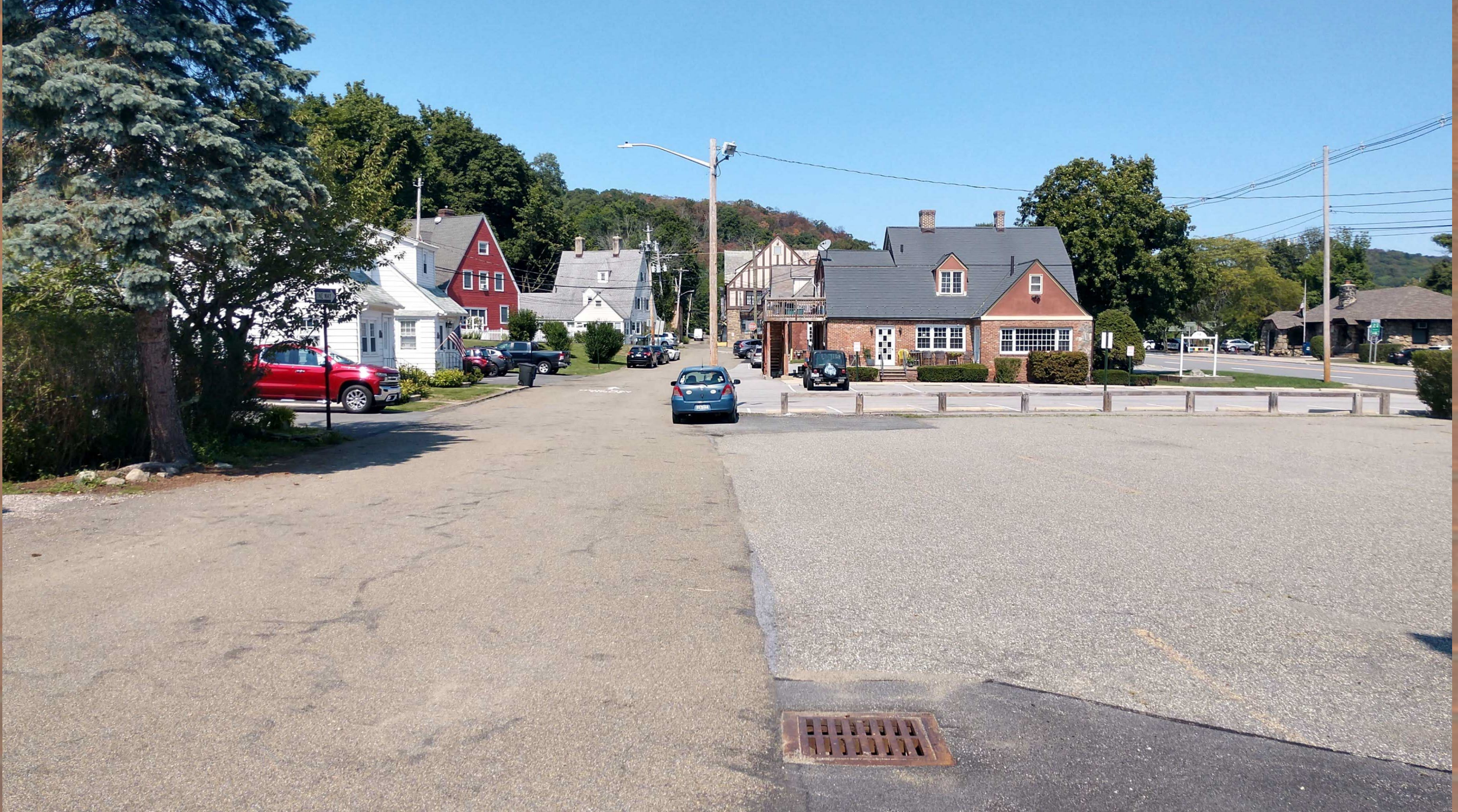
Figure 1: Store Road- existing conditions
