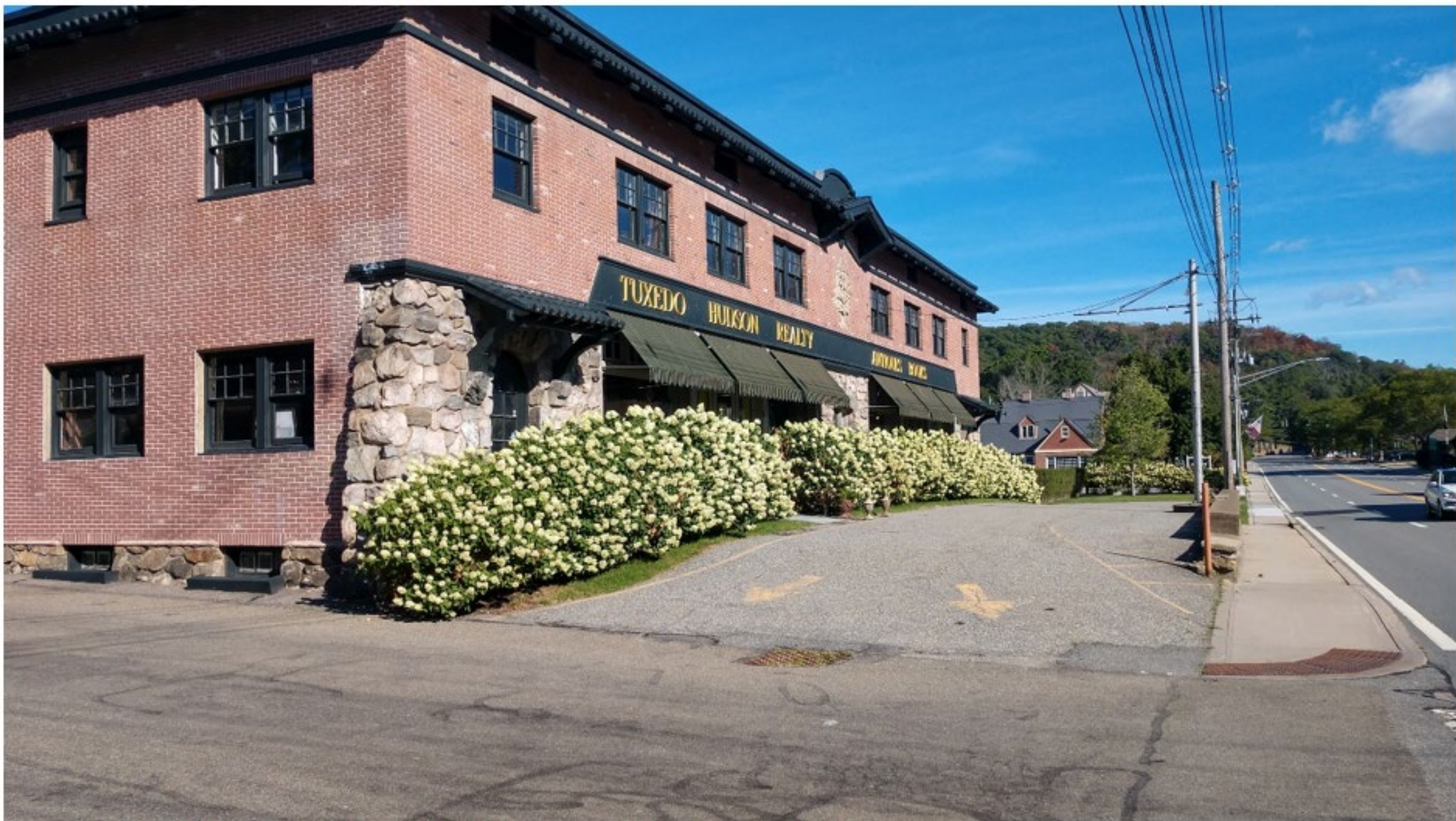
Image 12: Hospital Road intersection – adjacent driveway width existing conditions.
