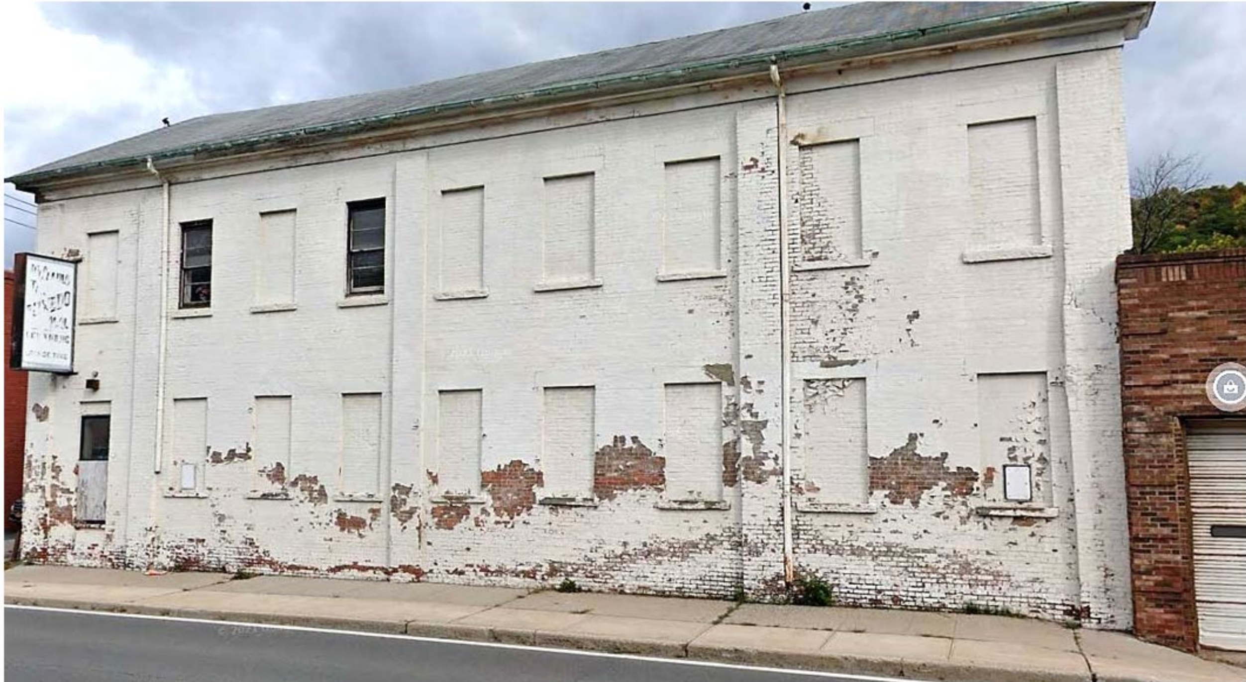
Figure 7: Existing warehouse wall condition (Photo courtesy of Google Streetview)
