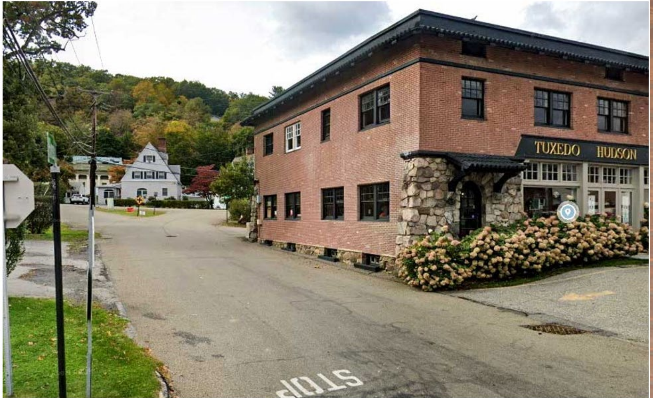
Figure 3: Hospital Road- existing conditions. (Photo courtesy of Google Streetview)
