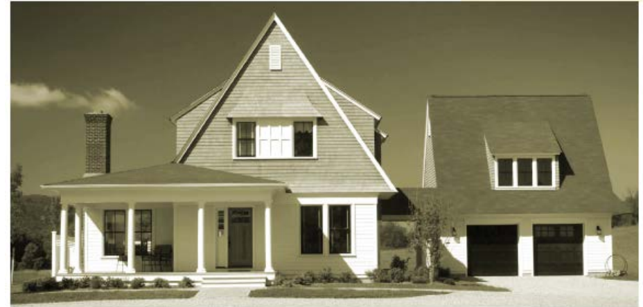
28.4 The garage is deferential to the main house by having a lower roof spring line than that of the main house. However, the two structures share similar materials and proportions, creating an aesthetic harmony among all parts.
